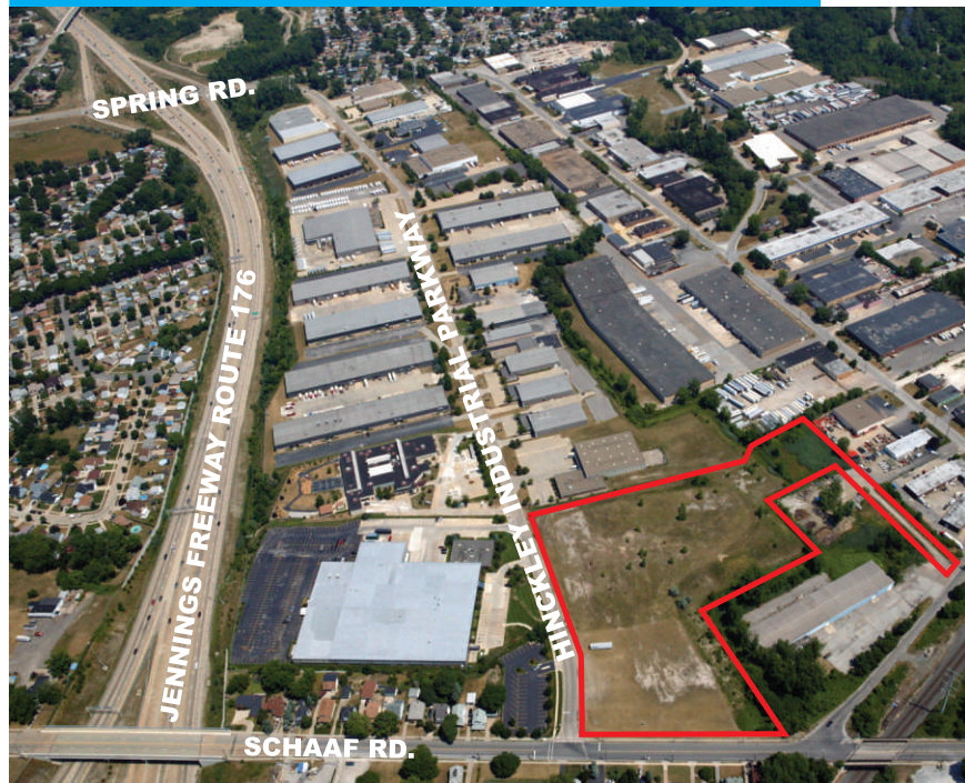
Office Site Jennings Freeway Industrial Park, Cleveland, Ohio
